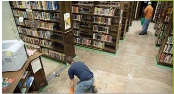
No harmful fumes, no building evacuation during installation.
